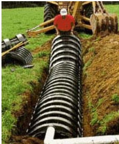
Figure 3. Example of pre-fabricated chamber (Infiltrator Systems, Inc.)
