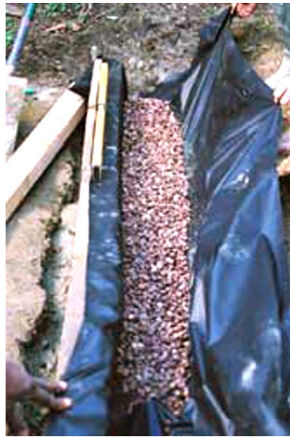
Figure 4. Construction of a French drain. ( www.gardenadvice.co.uk/howto/garden-build/frenchdrain/index.html )
